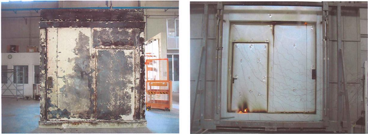
Fig.1: Standard fire test for one specimen barrier including a pass door– Exposed side (left side) and unexposed side (right side) after fire resistance test
